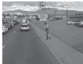
Existing Pedestrian Facility
