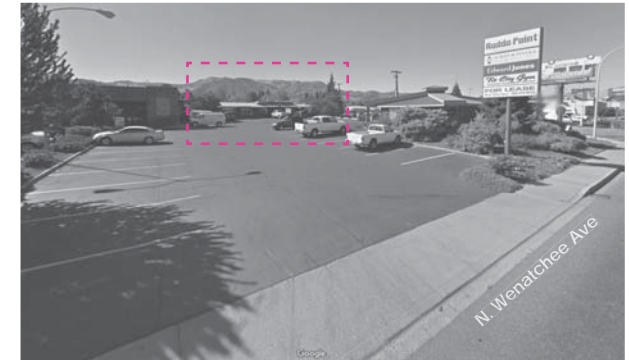
EXISTING: Medical Facility
