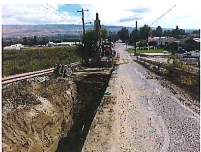
Excavating north side of Springwater
