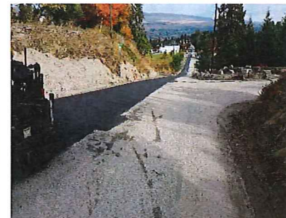
Final paving at Woodward
