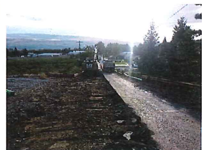
During construction facing east
