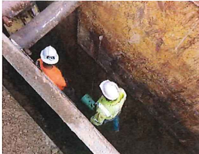
Installation of new sewer pipe
