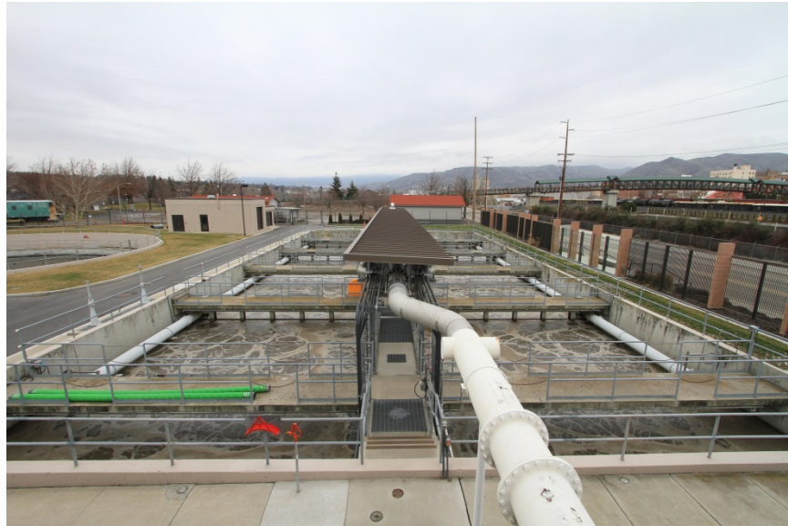
Figure 3-8. Existing Aeration Basins
