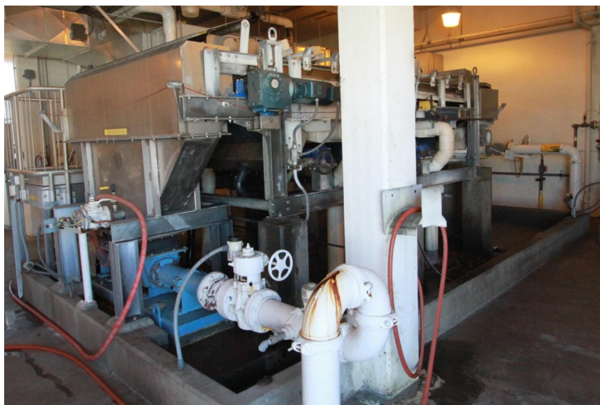
Figure 3-14. Gravity Belt Thickener
