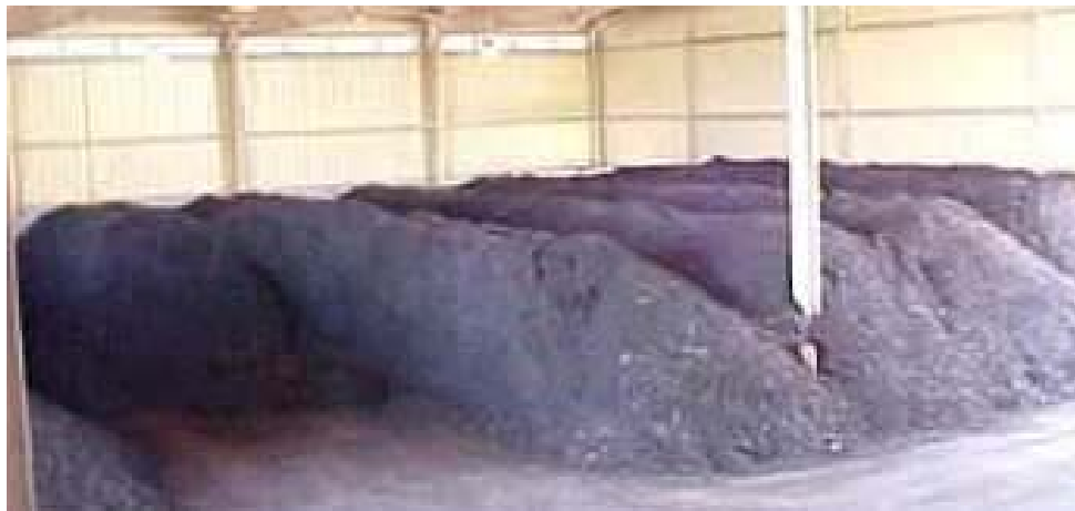
Figure 4-16. Example Aerated Static Pile Composting Facility (Coeur d'Alene, ID)
