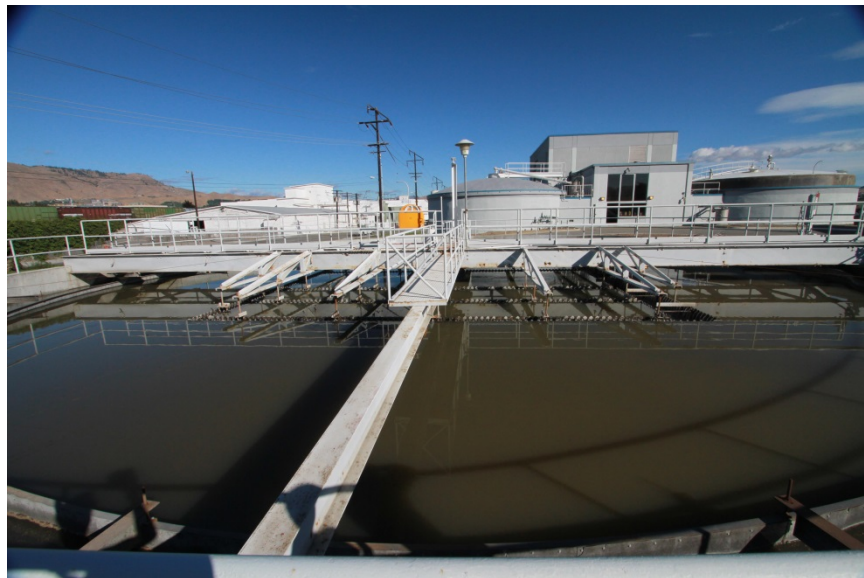
Figure 3-4. Existing 85 ft PCL before Odor Control Covers
