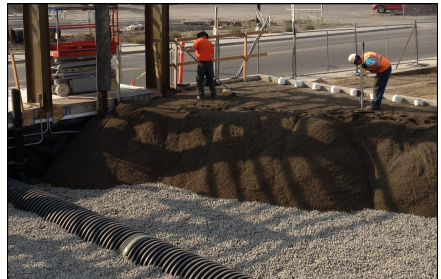
Installing the media in the biofilter
