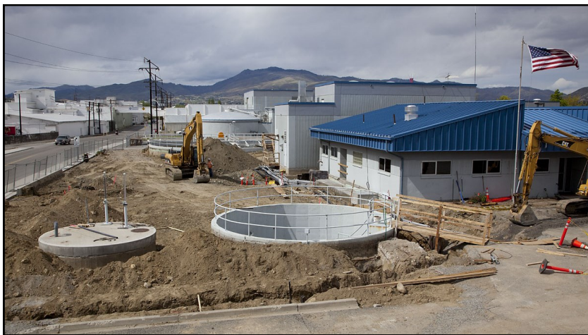
Construction started where the new Headworks building would be.
