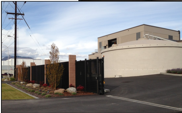
Landscaping and a new fence along Worthen Street
