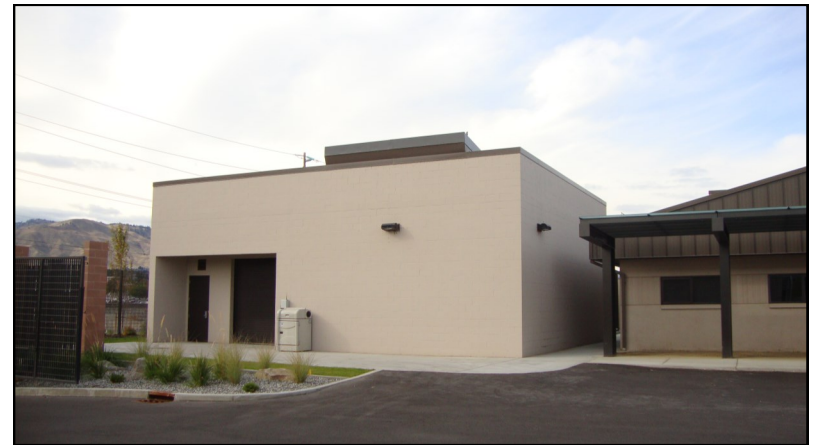
The completed Headworks Building
