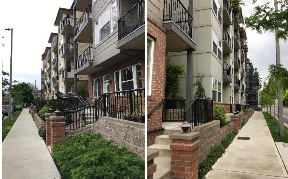
Figure C.1.c. The above images show ground-level residential frontages with setbacks of approximately 10 feet (left image) and 5 feet (right image) along different street frontages for this corner apartment building. These ground level units all have their own private unit access from the sidewalk and are elevated above the sidewalk to enhance the privacy to the units. The landscaping elements, brick posts, split-faced concrete block stoop walls, and black metal railings help to provide an attractive and effective transition between the public and private realm within the adjacent dwelling units.
