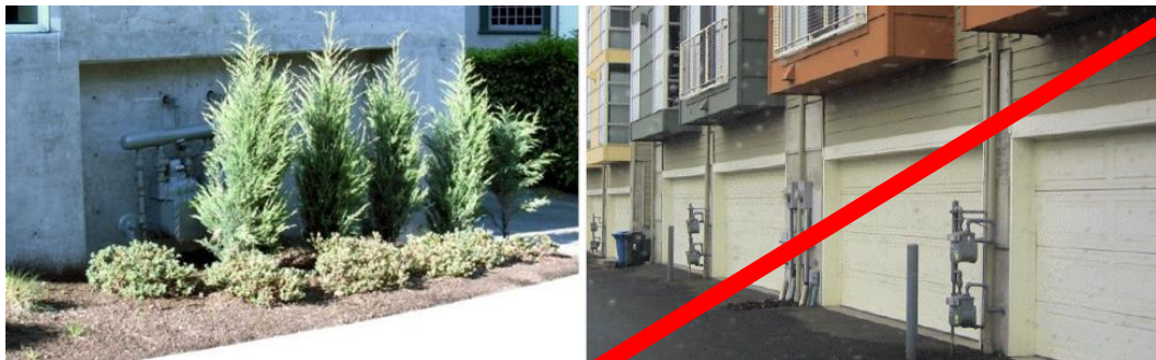
Figure C.7.4.a. Place utility meters in less visible locations. The left example successfully tucked the meters in a less visible location and/or screened by vegetation. The right example is poorly executed and would not be permitted in visible locations but may be acceptable on an alley or in a screened service area. Such meters must be coordinated and better integrated with the architecture of the building.
