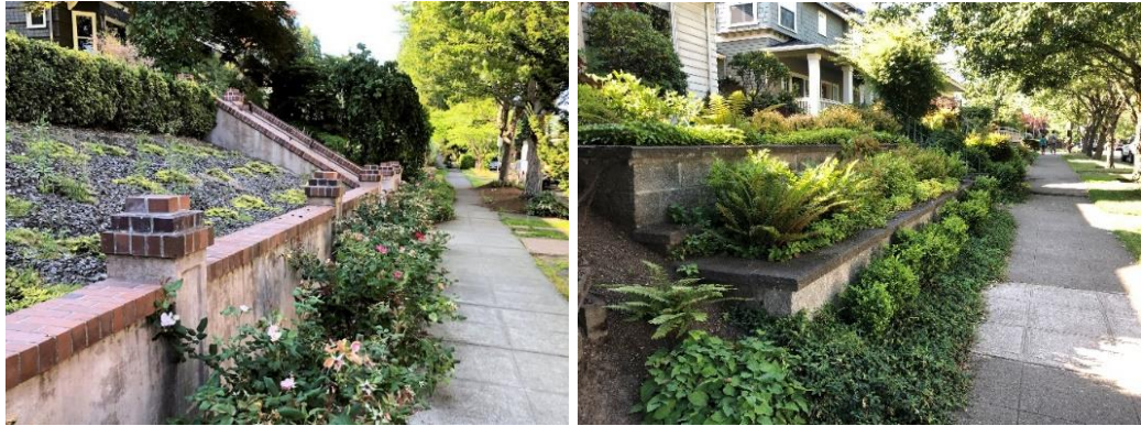
Figure D.5.1.d. Examples of appropriate measures to handle grade change in street front setbacks.
