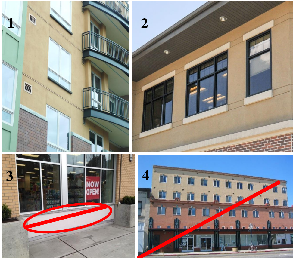
Figure E.6.1.e. Examples of acceptable and unacceptable use of EIFS. Buildings 1 and 2 mix EIFS with brick and other materials and integrate trim details around windows to add a sense of depth to the facade. Building 3 uses EIFS in between the window and sidewalk - this design is prohibited. Building 4 uses EIFS as the primary siding material, which is prohibited except in the North and South Wenatchee Business District areas.
