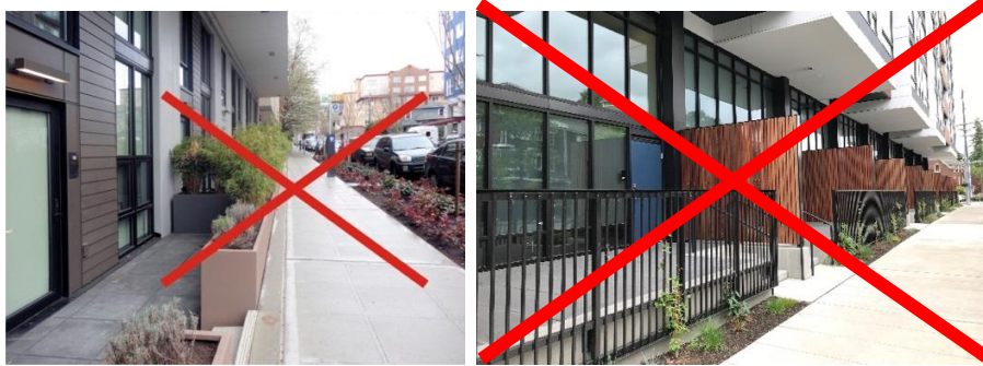
Figure C.1.d. Ground floor residential units such as these often lack privacy and the livability of outdoor spaces is limited. Locating the ground floor at or close to grade or with insufficient setback results in an uninviting space even with the planter in place. This condition should be avoided.
