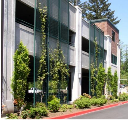
Figure E.8.1.a. The side of this parking garage includes decorative grillwork and a raised brick planter to enhance the pedestrian environment.
